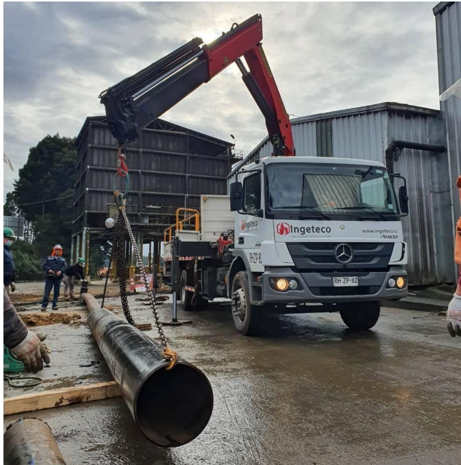
6x2 6m Truck Crane (5.4-ton crane with 12-meter extension)
